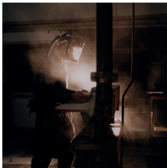
Figure 4b Photograph showing dust cloud from the sanding operation
